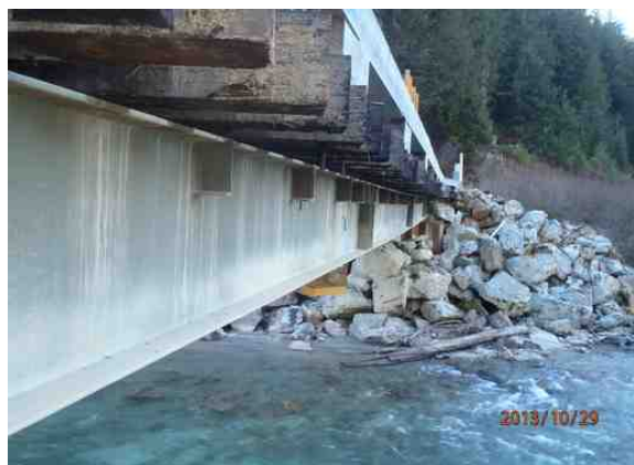
Figure 1-9: Upstream girder- viewed from left abutment.
