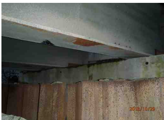
Figure 1-21: Right abutment sill.
