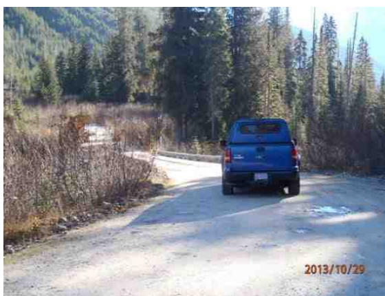
Figure 1-5: Right approach - looking toward bridge.
