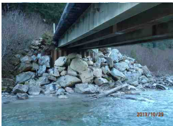
Figure 1-19: Right abutment face.
