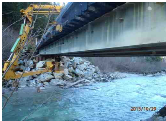
Figure 1-10: Downstream girder- viewed from left abutment.
