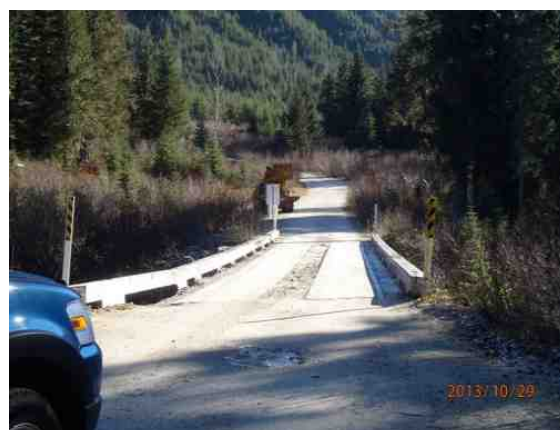
Figure 1-6: Left approach- looking toward bridge.
