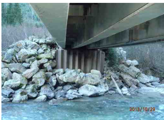
Figure 1-23: Left abutment face.
