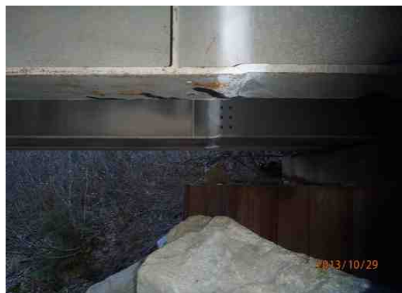
Figure 1-16: Offset butt welds at right abutment.
