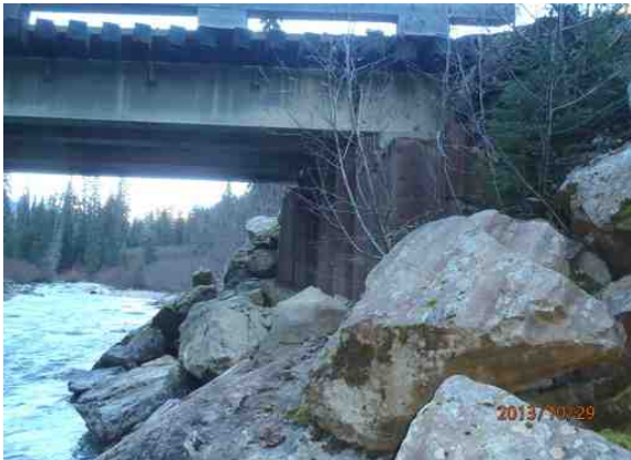
Figure 1-27: Left abutment - rip rap.
