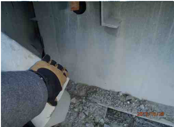
Figure 1-25: Left abutment- upstream bearing.
