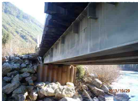
Figure 1-8: Upstream girder viewed from right abutment.
