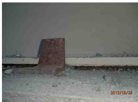
Figure 1-24: Left abutment-bearing at girder #4.
