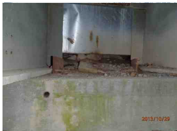
Figure 1-20: Bearings at right abutment.
