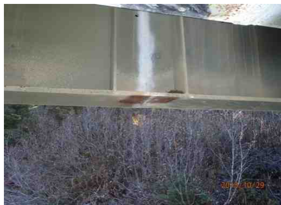
Figure 1-12: Previously inspected butt weld.
